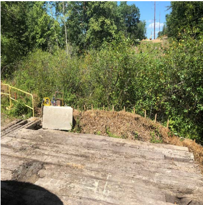
Fig 19: Erosion controls between Str. 28 and Oyster River. Viewing north. (8-20-19).
