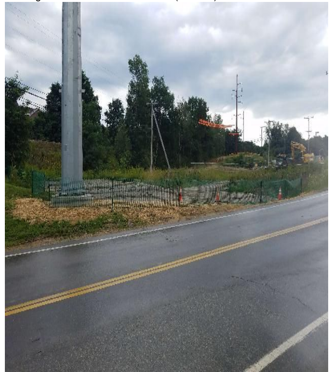
Fig 24: Green pedestrian fence installed around Str. 24 work pad. Viewing southeast. (8-21-19).
