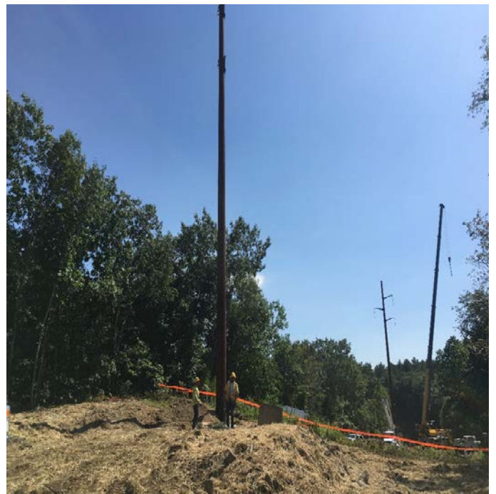
Fig 4 JCR installing Strs. 26 and 27. Viewing south. (8-15-19).
