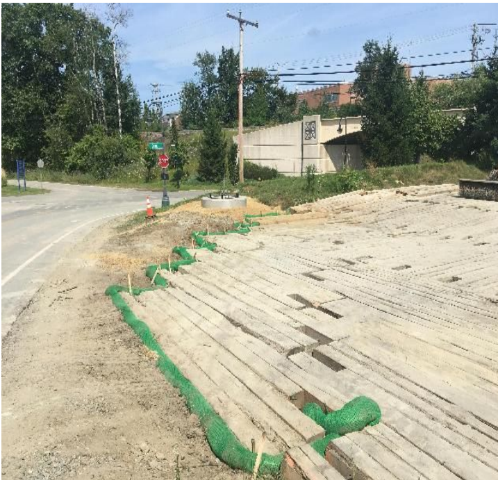
Fig 7: Str. 24 work pad with erosion controls. Viewing north. (8-16-19).
