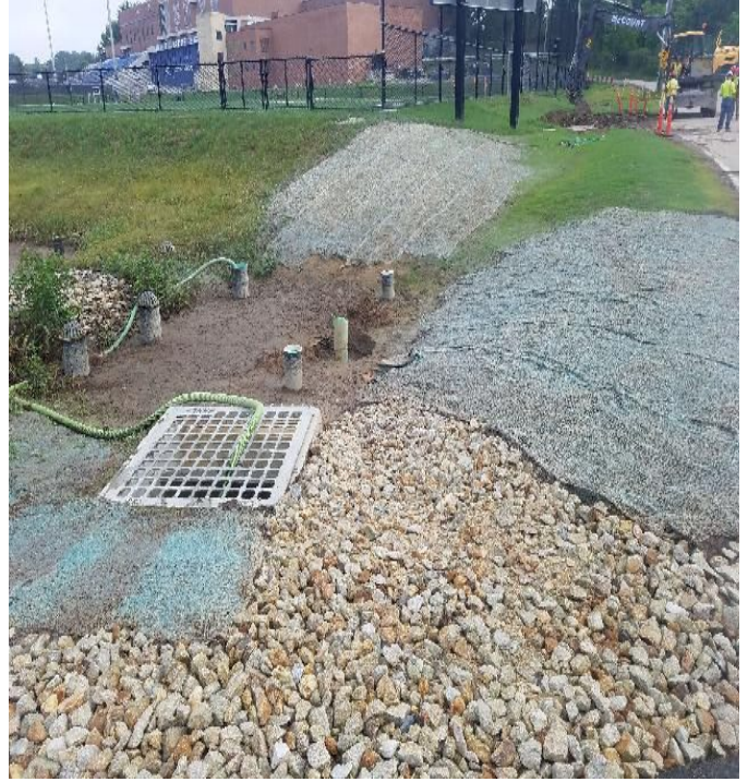
Fig 14: Rain garden restoration and hydroseed. Viewing north. (8-19-19).
