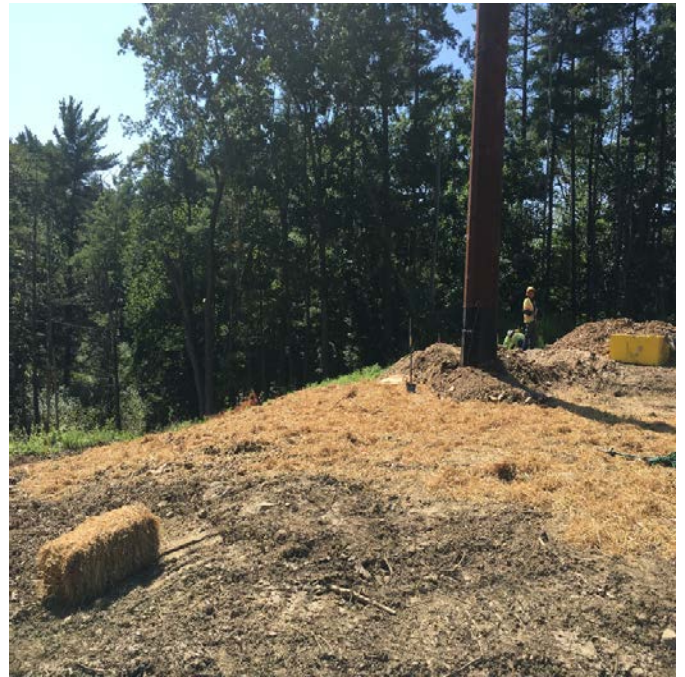
Fig 2: Spreading straw on exposed soils around Str. 27. Viewing southwest. (8-15-19).
