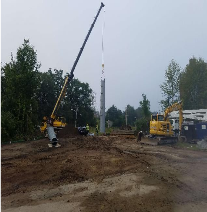
Fig 13: JCR beginning to construct Str. 23. Viewing south. (8-19-19).
