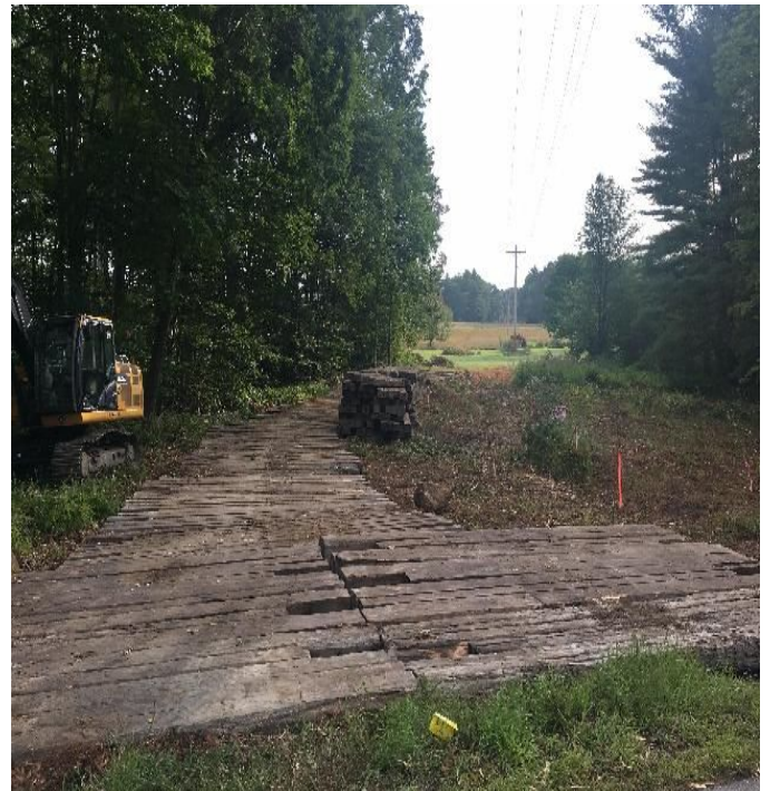
Fig 20: Fox Point Rd access. Viewing northeast. (8-21-19).
