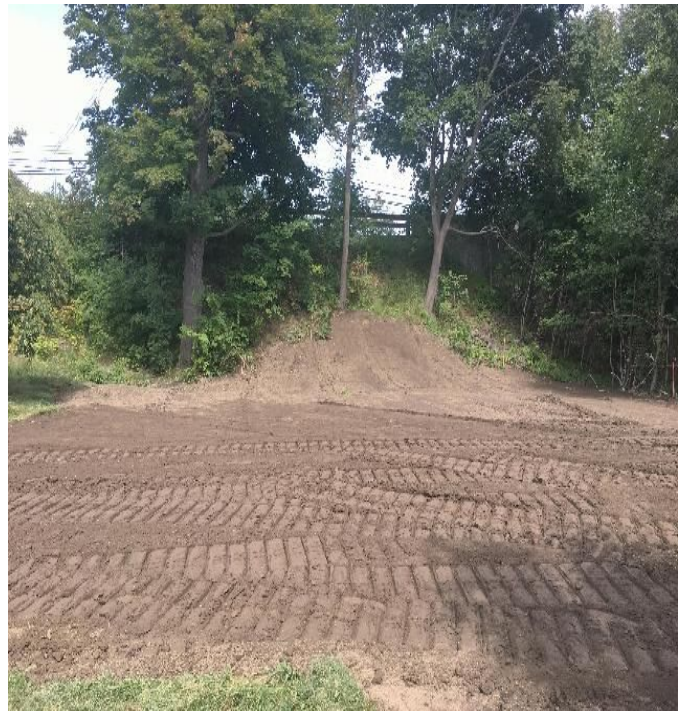
Fig 6: Restoration of receiving pit next to UNH field house. Viewing north. (8-16-19).
