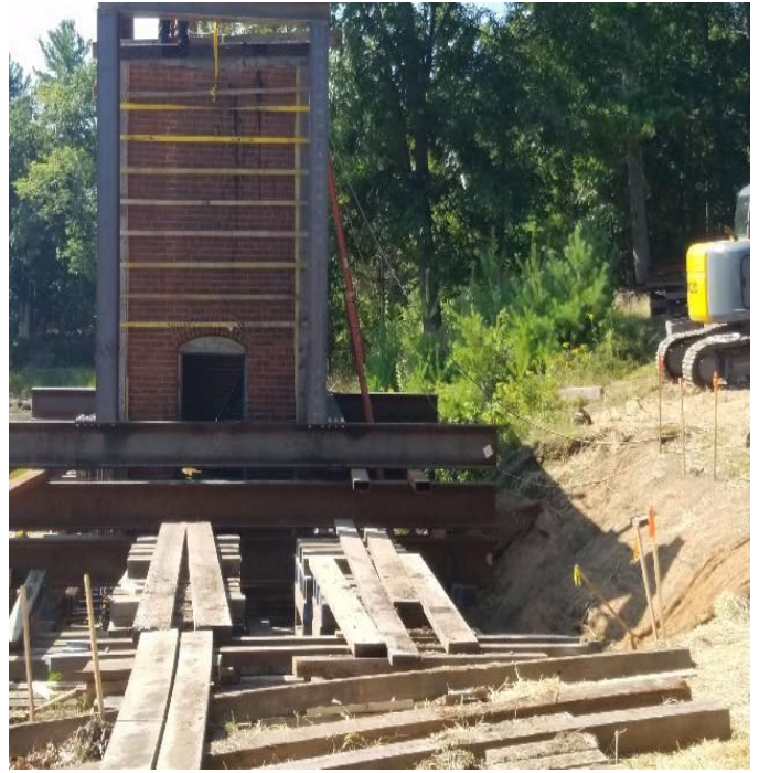
Fig 10: Cable house progress. Viewing south. (8-16-19).
