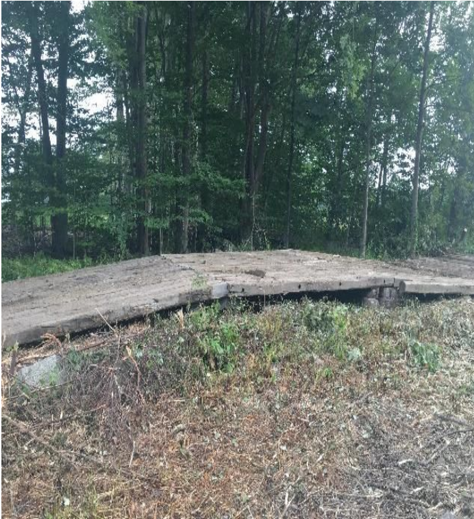
Fig 21: Elevated timber mat over stone wall WP-45. Viewing north. (8-21-19).
