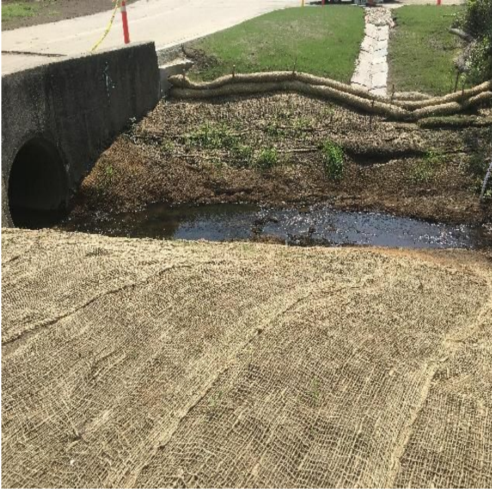
Fig 5: College Brook restoration. Viewing south. (8-16-19).
