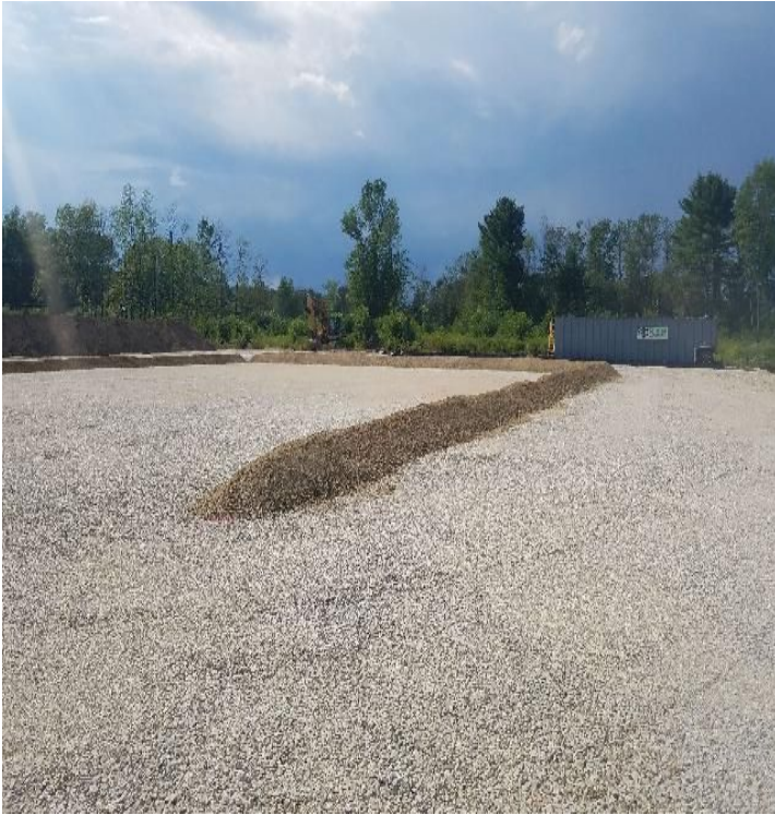
Fig 17: Shattuck road laydown area progress. Viewing north. (8-19-19).
