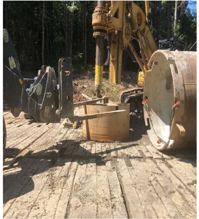
Fig 18: Prepping to drill Str. 28. Viewing west. (8-20-19).
