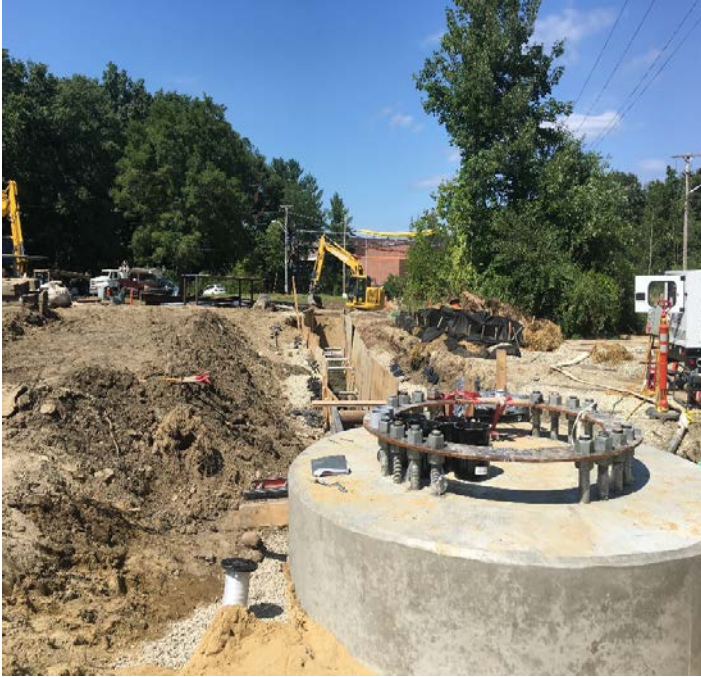
Fig 1: McCourt trenching towards Str. 23. Viewing north. (8-15-19).
