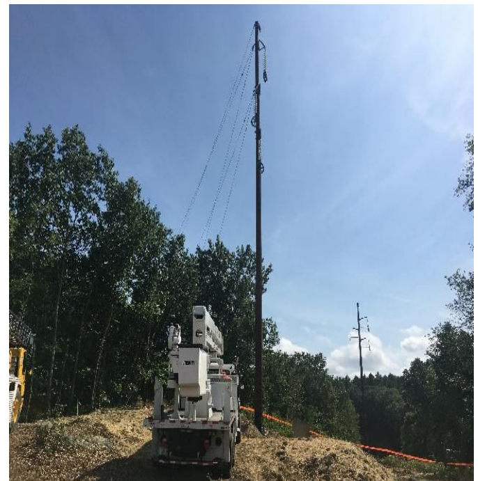
Fig 8: Str. 26 installed. Viewing south. (8-16-19).
