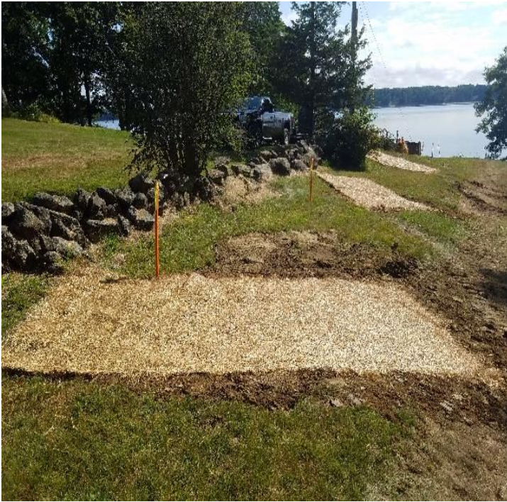
Fig 9: Test pit locations at the cable house. Viewing east. (8-16-19).
