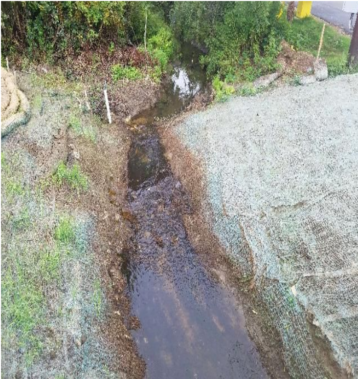
Fig 15: College Brook restoration with hydroseed on the slopes. Viewing west. (8-19-19).
