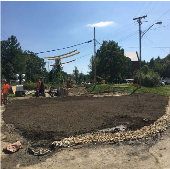
Fig 3: Underground cable corridor at intersection of Colovos and Waterworks Viewing south. (8-15-19).
